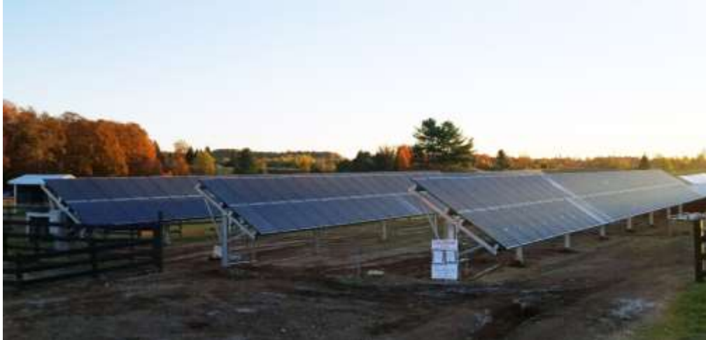
Figure 1 - Photograph of the solar arrays positioned by the petting zoo and livestock area
